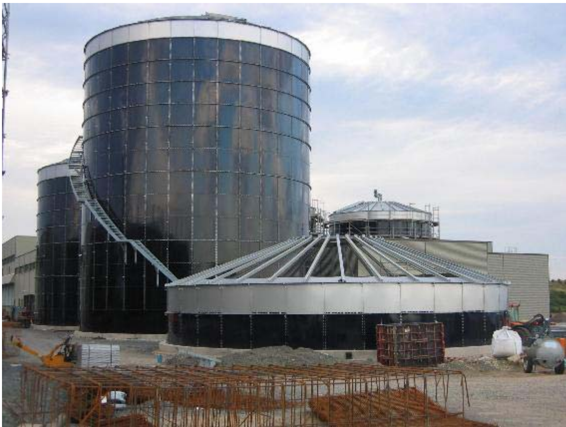
Figure 1. The three fermenters during the construction phase (Abfallzweckverband Südniedersachsen, 2005).
